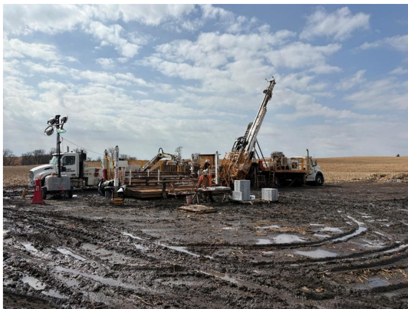
Figure 10-2 Drilling in progress at Rift Rare Earth Project – RIFT26-006 and RIFT26-005A
